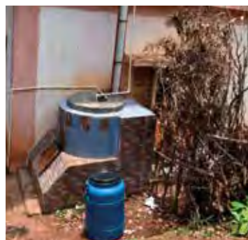
Dry waste incinerator for hot water and bio-gas for cooking at D. Modhaputtu Ashram School Complex
