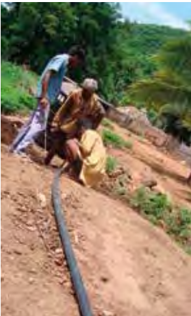
Gravity flow mechanism for channeling water to Munagalapudi village
