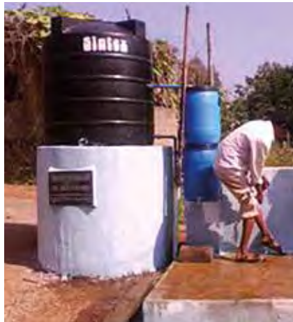
Gravity flow mechanism for channeling water to Munagalapudi village
