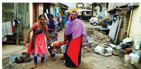
Figure 6. Slum residents constructing their toilet.
