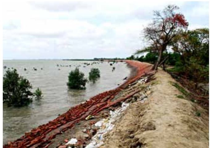
Broken river bund, Brajaballavpur, Patharpratima
